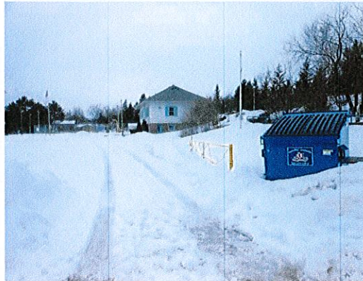
Photo 2: There is an on-grade entry to the upper and lower levels. There is not an interior accessible route between levels (stairs only).
