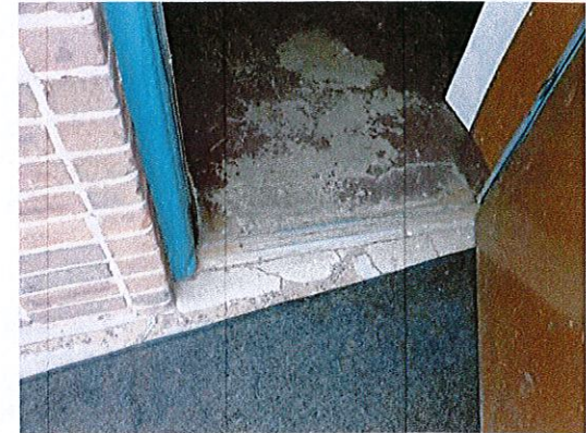
Photo 3: Patch the threshold at the lower level entry.
