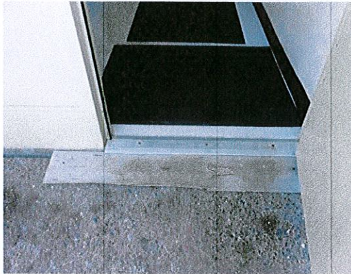
Photo 2: Replace the wood transition at the threshold.
