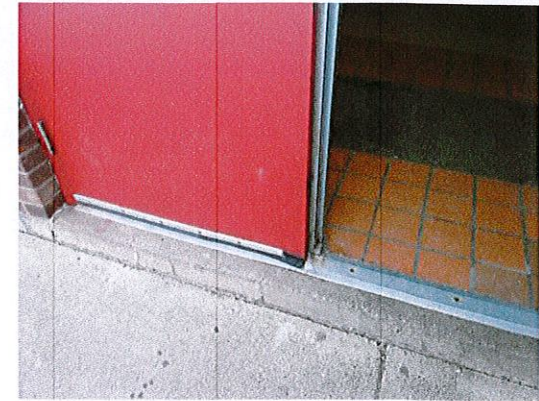
Photo 3: Eliminate the 6" rise at the SW entry. (This is the primary entry used by ECFE staff.)
