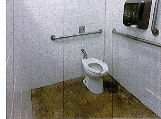
Photo 3: The toilet rooms currently provide features of accessibility. Relocate the toilet paper dispenser to below the side grab bar.
