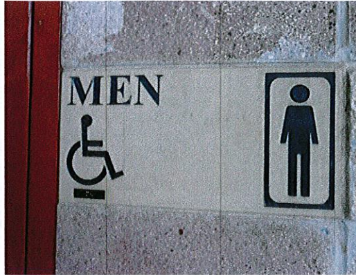
Photo 2: The signs currently provide braille, but do not have raised characters (they are engraved).
