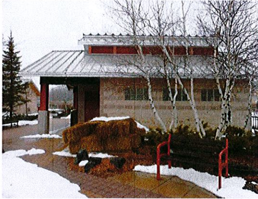
Photo 1: An accessible route is provided to the bathroom building. This is a good example of accessibility.
