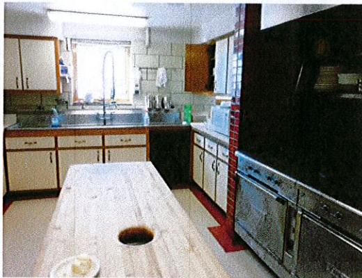
Photo 4: View of kitchen. There are currently no features of accessibility provided. (Commercial appliances are provided, but this is not a commercial kitchen.)
