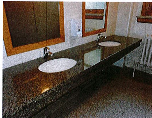
Photo 11: Remodeling in the 1st and 2nd floor toilet rooms incorporated accessibility- such as providing sinks with knee and toe clearance and easily operable faucet hardware. This is a good example of accessibility.
