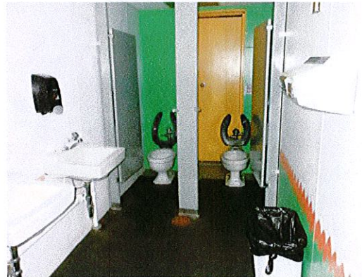
Photo 11: The lower level toilet rooms currently provide no features of accessibility.
