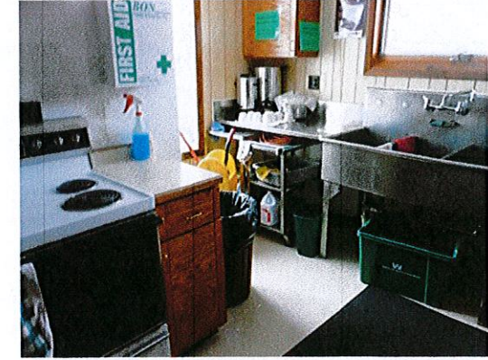
Photo 6: View of kitchen. There are currently no features of accessibility provided.
