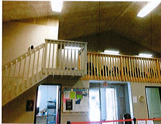
Photo 5: A small viewing loft is provided in the gymnastics area. There is not currently an accessible route. Add handrails at the stairs.
