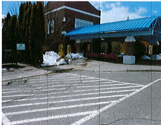
Photo 2: Patch and repair the curb cut.
