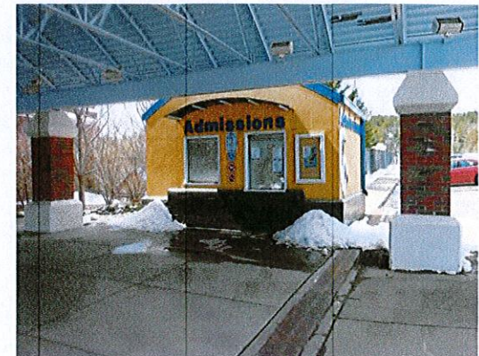
Photo 3: The ticket windows at the exterior admission building are currently at 37" (vs. 36" maximum).
