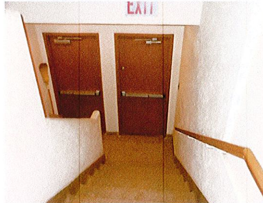
Photo 2: View of main entry. There is not an accessible route to the upper level. (The lower level has an on-grade entry.)
