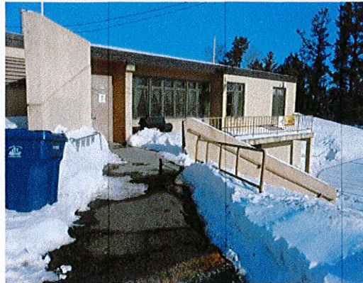
Photo 2: There is an on-grade entry to upper level from the parking lot. There is not currently a route to the lower level. (There is no interior route between the 2 levels, only exterior stairs.)
