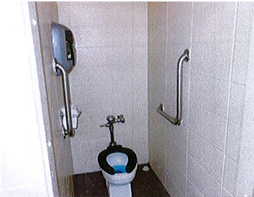
Photo 4: An ambulatory accessible stall has been provided, but not a 5' wide stall.
