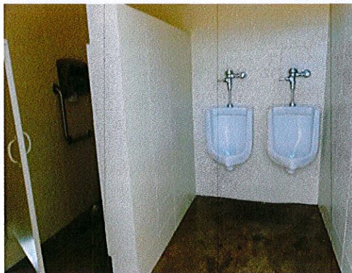
Photo 5: Lower 1 of the urinals to 17" max (currently at 24").
