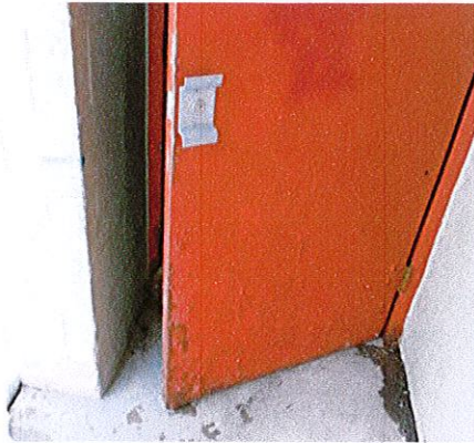
Photo 1: Maneuvering clearance is not currently provided at the entry door.
