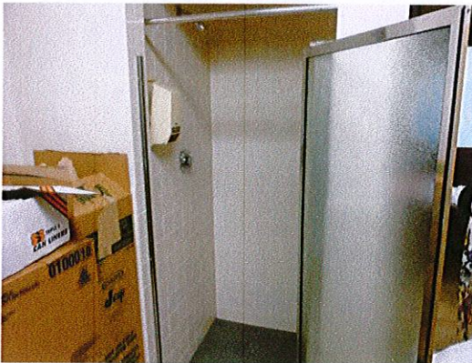
Photo 4: View of shower. The shower does not currently provide seat, grab bars or hand held shower wand.
