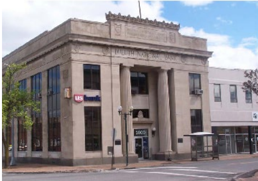
Example of Corridor Building II
