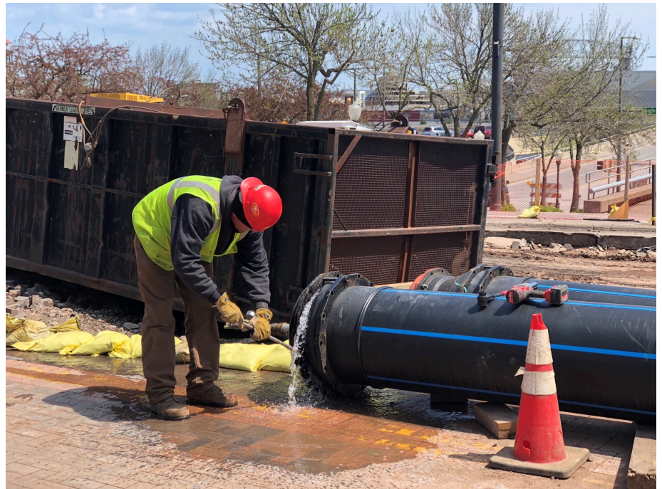
testing the permanent watermain
