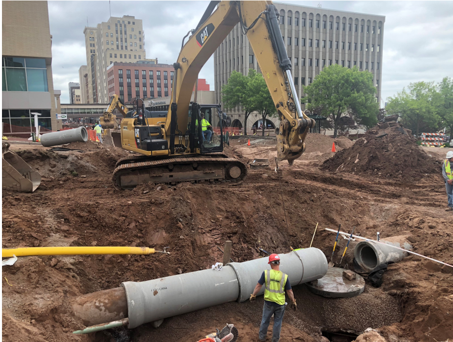
stormwater pipe installation
