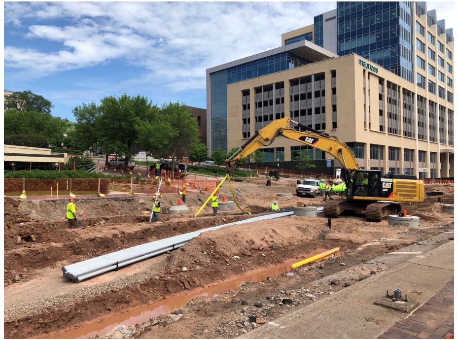
Ongoing work at 5th Ave W - Electrical ducts piled for installation
