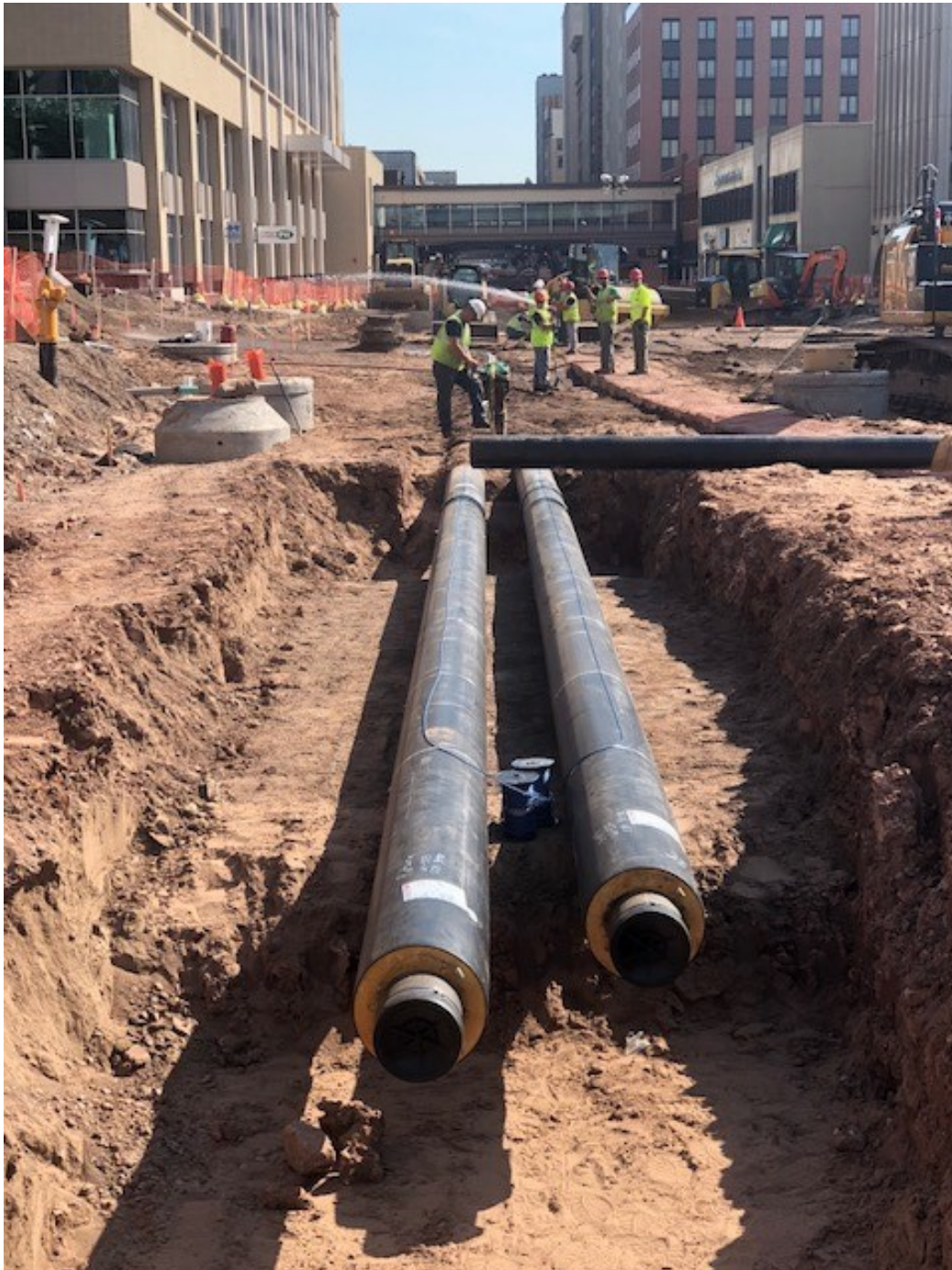
hot water lines installed
