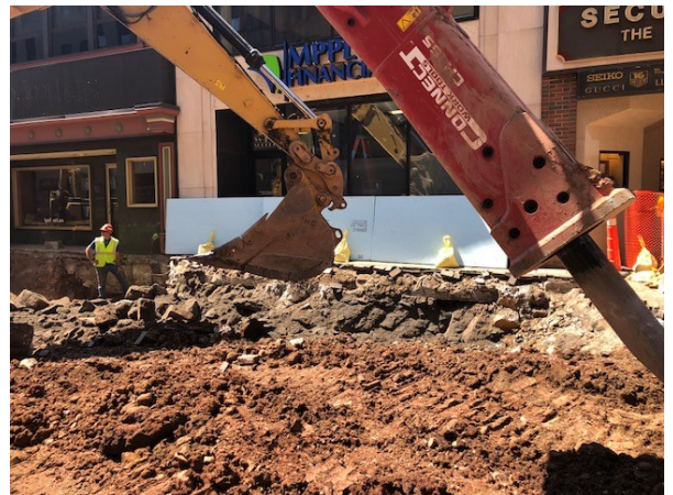
Preparing to install new water into MPPL Financial building
