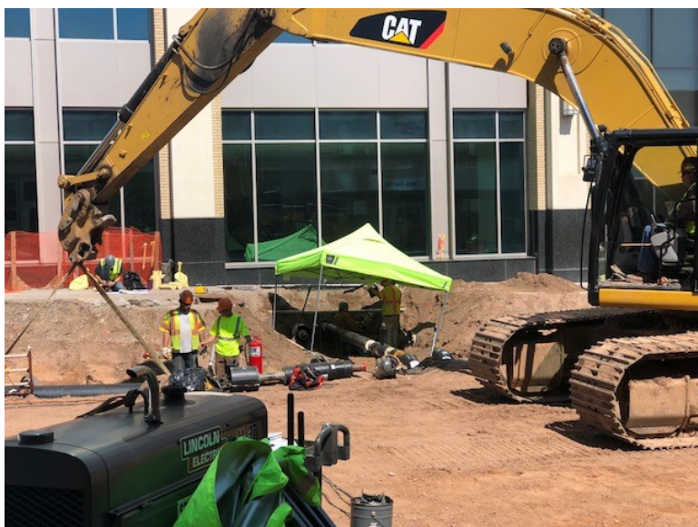
Crews installing hot water to maurices
