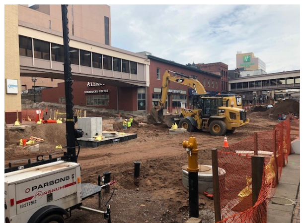
Excavation of 4th Ave West for hot water installation
