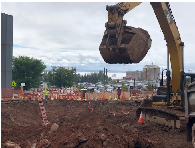
Crews preparing for utility installation on 6th Avenue W.
