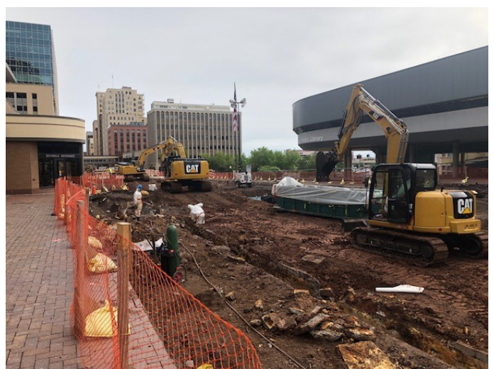
Removal of the last of the 100 year old steam line in front of the Radisson
