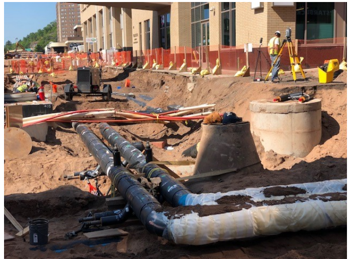
Hot water pipe installed on 4th Avenue W.
