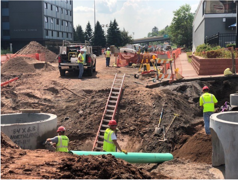
Storm water pipe installation
