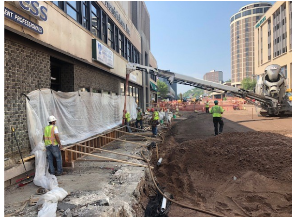
pouring concrete into the vault at Northland Building
