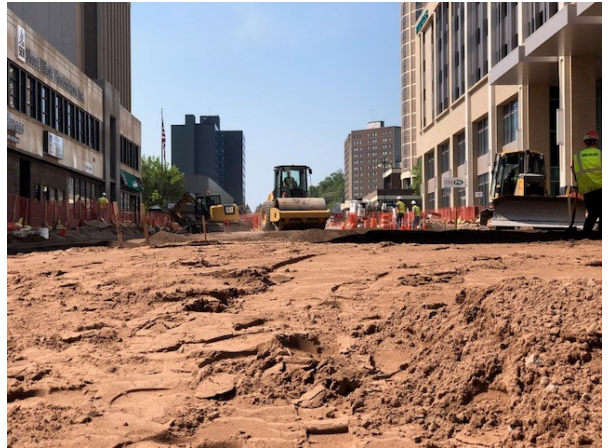
prepped for concrete in the coming weeks
