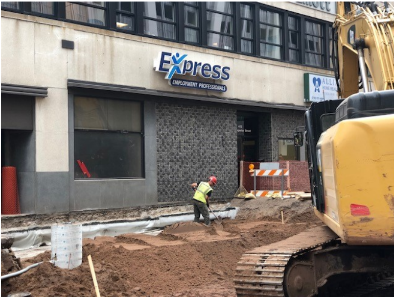
back filling the vault in front of Northland Constructors
