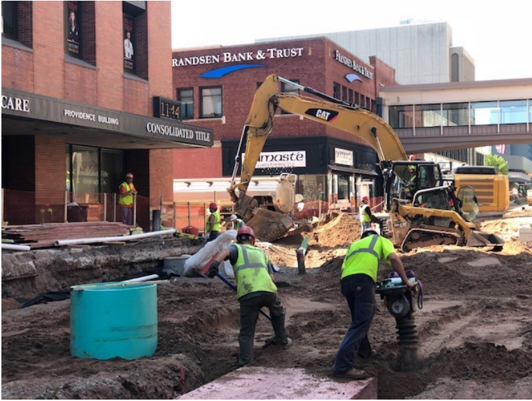
Work on 4th Ave West -tamper in action
