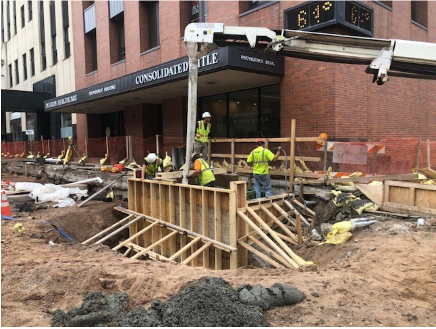
work on a vault and signal base
