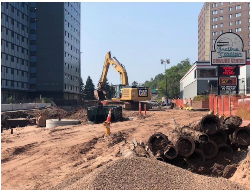
installing the last water main
