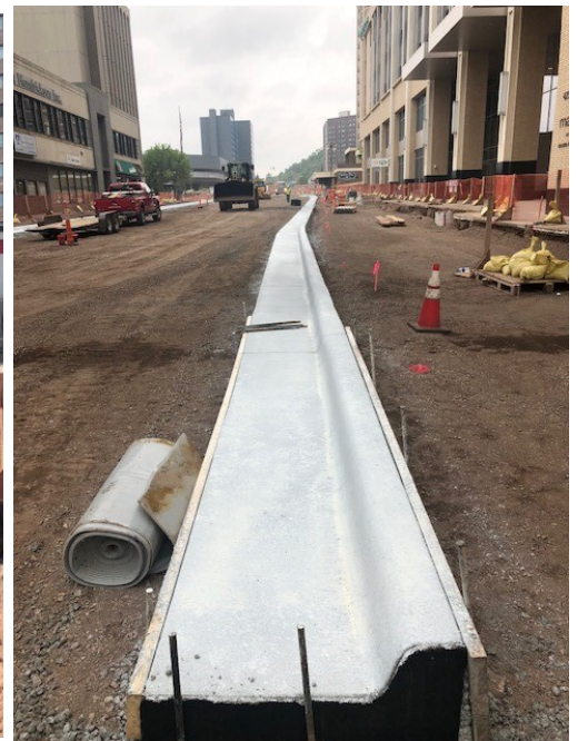
curb and gutter up close
