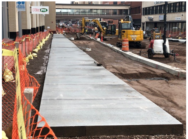
sidewalk poured in front of maurices
