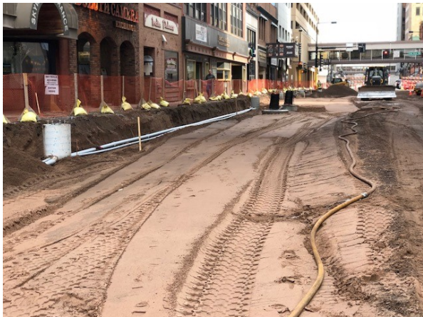
graded road ready for concrete
