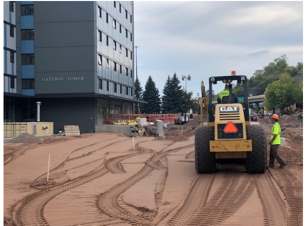
preparing the road for concrete by Gateway Tower
