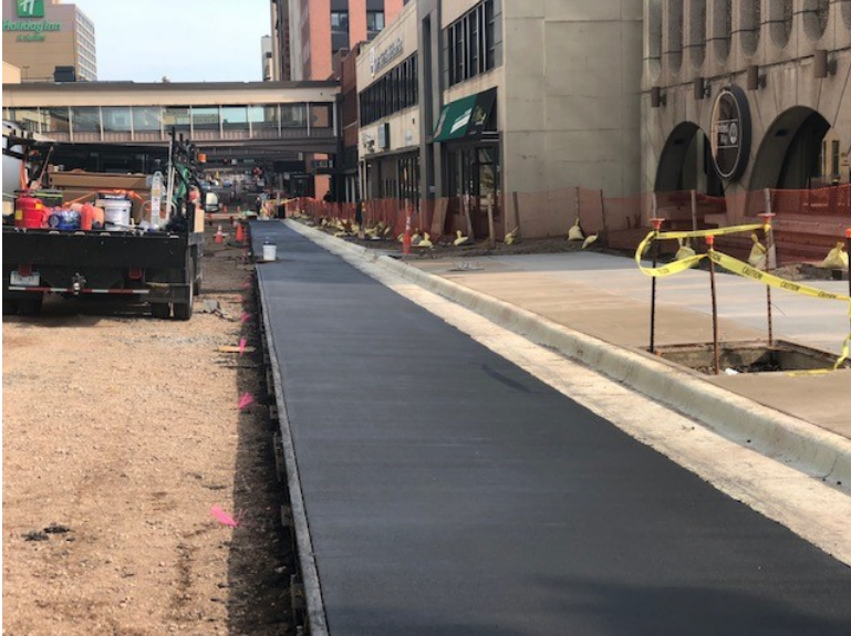
New parking lanes installed between 3rd and 4th Ave West
