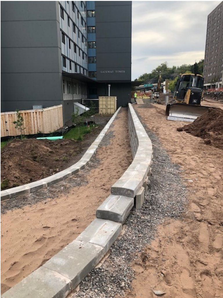
New retaining wall installed by Gateway Tower
