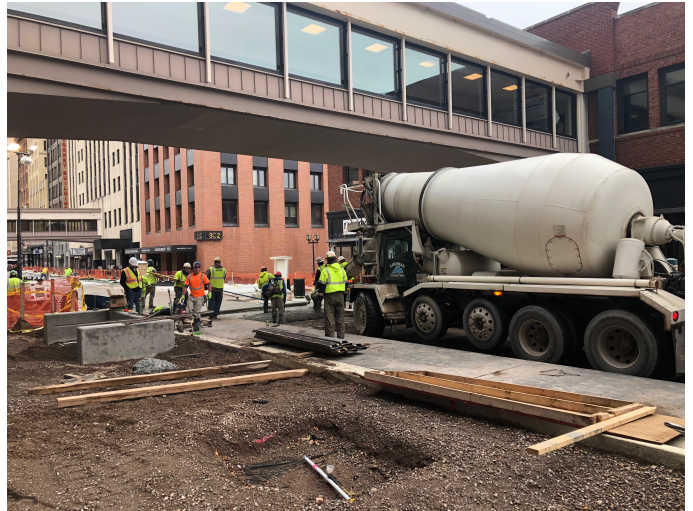
crews pouring concrete for the driving lane between 4-5th Ave W
