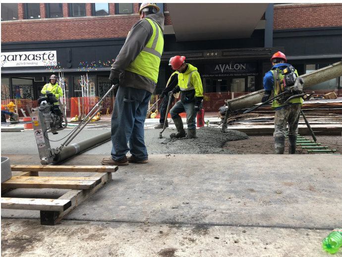
Crew smoothing out concrete between 4-5th Ave W
