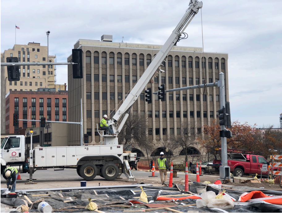
Installing traffic signals
