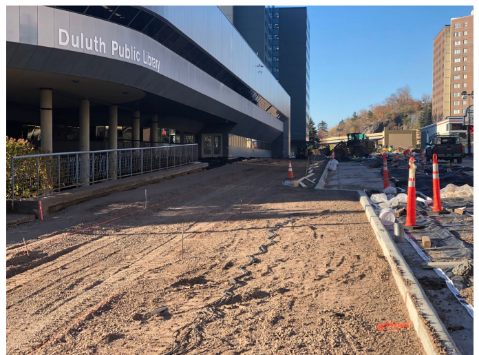
soil compacted for new sidewalk installation
