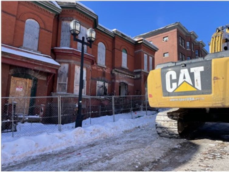
Contractor machinery arrives at site
