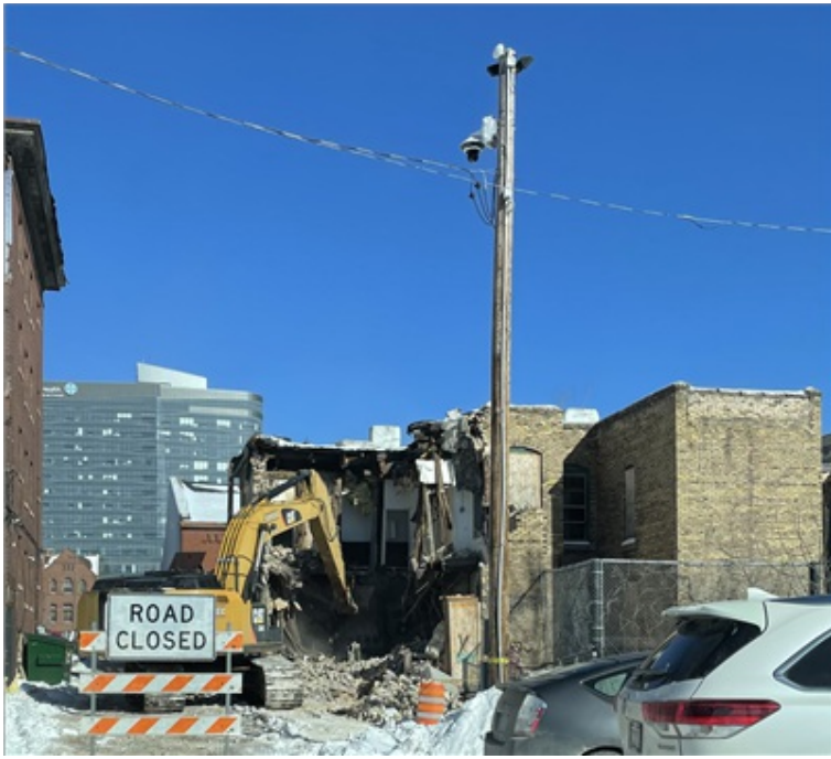
Rear corner demolition efforts
