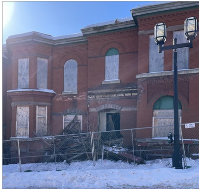
Street-level areas to be demolished
